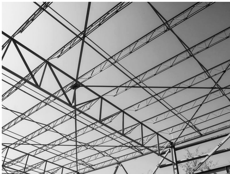
Figura 112. Sistema joistec. (Archdaily, 2014)
