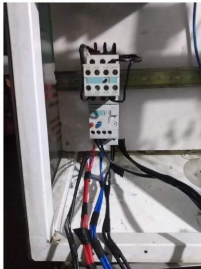
Figura 4-36: Contactor de 40 amperios
