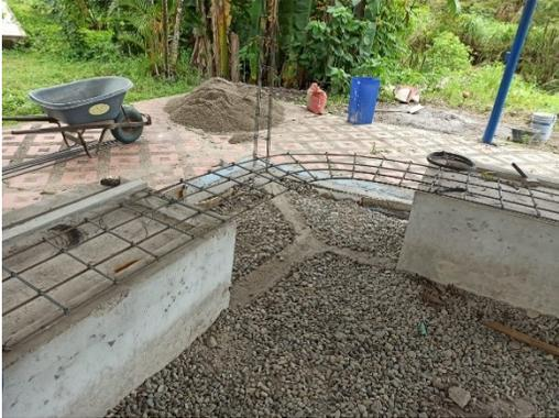
A photograph showing the construction of a concrete structure, likely a bench or seating area. The structure is made of concrete blocks and is surrounded by gravel. A wheelbarrow and other construction materials are visible in the background. | Alistamiento del lugar, construcción de la primera fila de gradas. |
