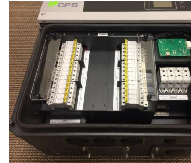
Figure 9-1. Remove Wirebox Cover
