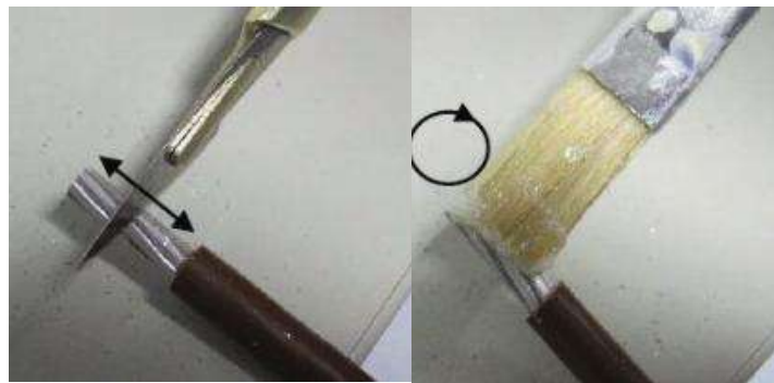
Figure 3-38 Preparing Aluminum Conductors prior to connecting
