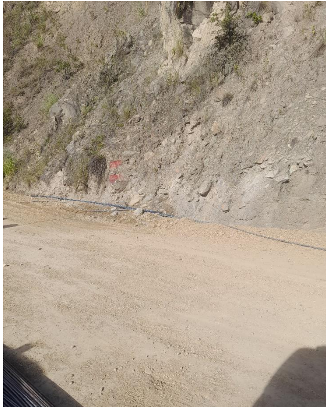
Figura 43 Sub base granular compactada
