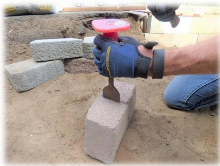
Ilustración 3. **Corte adoquín con cincel.** Fuente: Buckles, R. (2021). How to Lay a Retaining Wall with Concrete Blocks. The Spruce. <https://www.thespruce.com/lay-a-retaining-wall-with-blocks-1821048>
