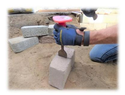
Ilustración 3. *Corte adoquín con cincel.* Fuente: Buckles, R. (2021). How to Lay a Retaining Wall with Concrete Blocks. The Spruce. https://www.thespruce.com/lay-a-retaining-wall-with-blocks-1821048
